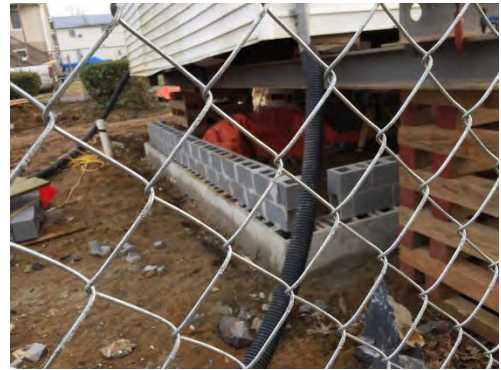
The renovated foundation
