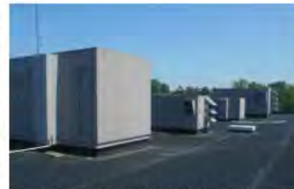
720-18576-94-01 VCBR RTUs (rooftop units) replacement
