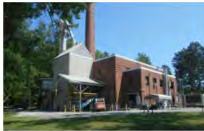
720-18576-29-11 PGH Boiler Plant upgrade
