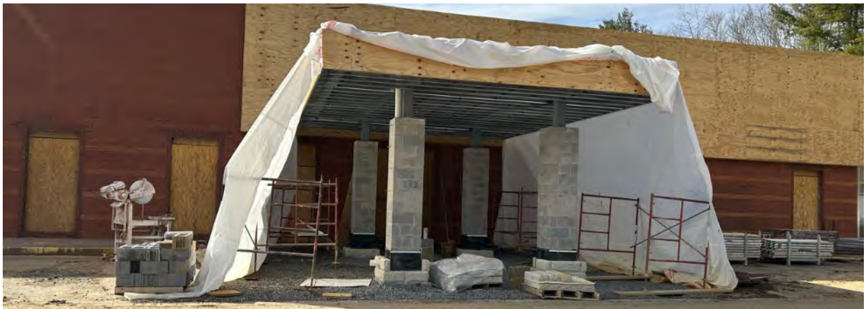
Actual Main Entrance Under Construction
