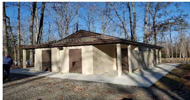
After photo – After the campground renovation. The campground and bathhouse at Westmoreland State Park is a very popular destination and needed renovations for maintenance needs and to make the bathhouse more accessible and family friendly. Campgrounds provide a low-cost choice for Virginians to enjoy overnight accommodations in an outdoor recreation setting like a state park
