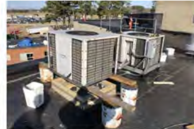
720-18576-29-02 PGH HVAC replacement
