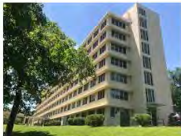
720-18576-24-02 Catawba Hospital HVAC replacement
