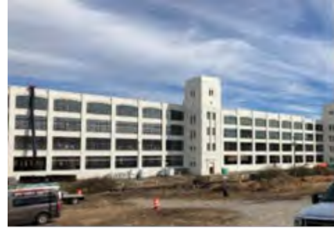
IRF ARPA provided $5 million for the redevelopment of the 600,000 sf “white mill” in Danville, Virginia into a mixed-use property.
