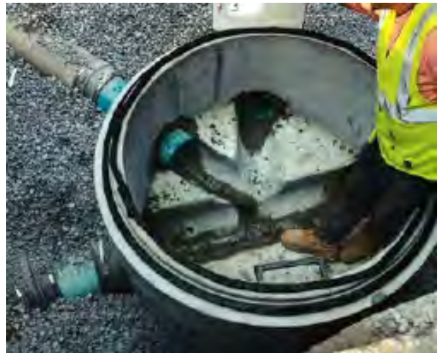
Nelson County (4400214): Manhole LR-38 being installed.
