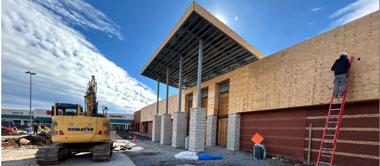
Actual Regional Workforce and Child Development HUB Main Entrance Under Construction
