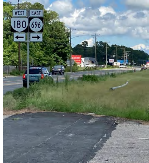
Hampton Roads Sanitation District (4400205): Force main installation and road crossing on the Eastern Shore.
