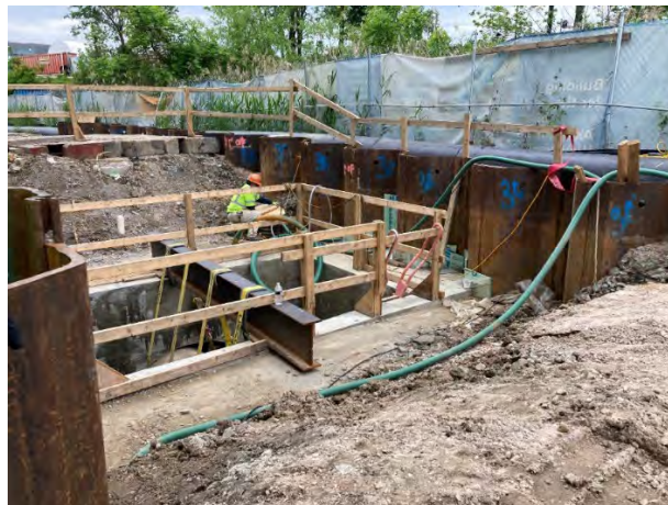
Alexandria Renew Enterprises (4400101): Diversion chamber under construction at Hoofs Run AAHP.
