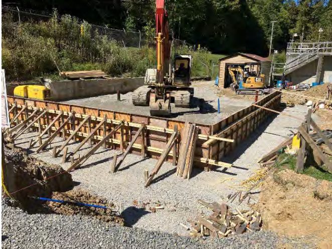
Wise County PSA (4400301): Sludge dewatering building construction.
