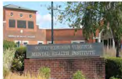
720-18576-05-01 SWVMHI HVAC replacement
